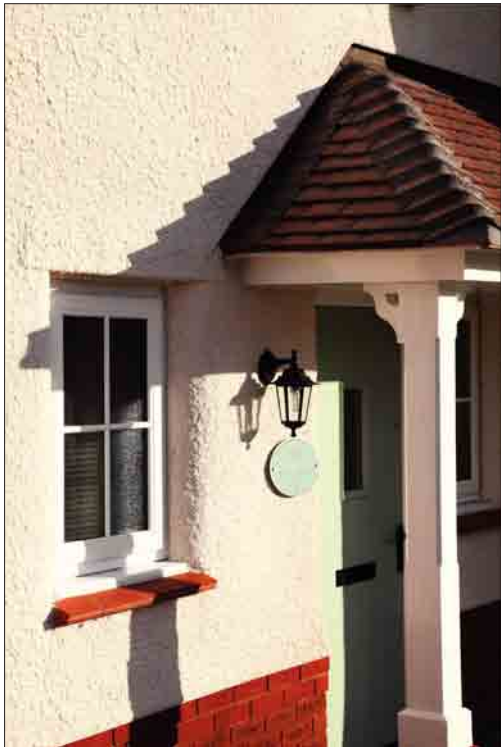
Photo 6 : Timber post porch
