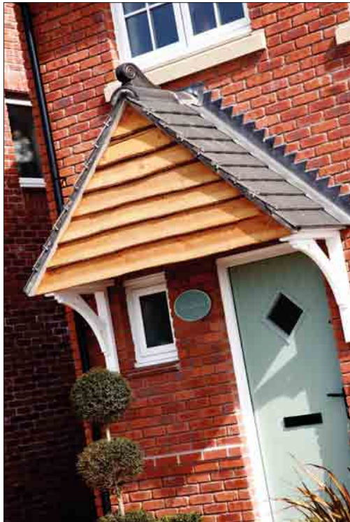
Photo 5 : Wavy edge boarding on porches
