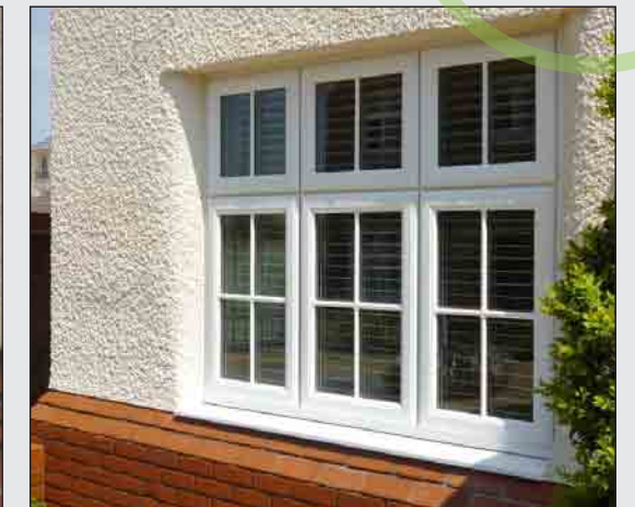
Photo 9 : Roughcast white render rounded into the window reveal
