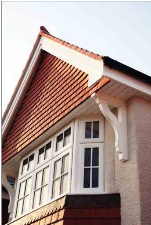
Photo 3 : Tile hung gable end
