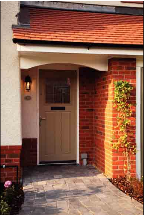
Photo 7 : Tile roof porch
