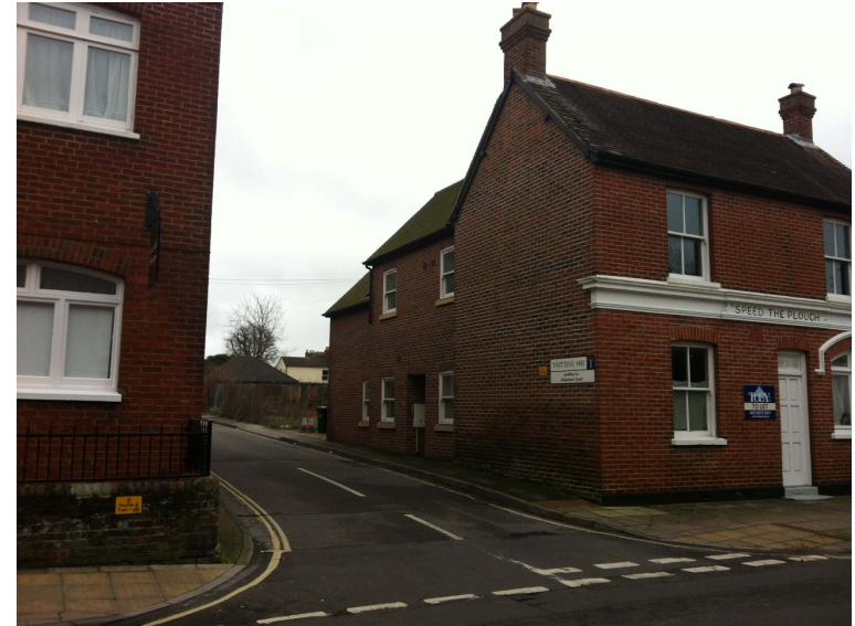
Image 7: Photo showing the entrance to Twittens Way from South Street
