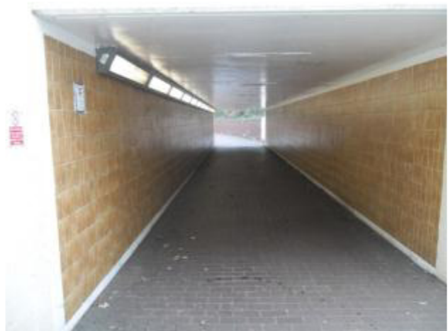
Photo 3.6: Maurepas Way underpass
