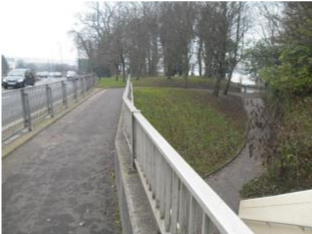
Photo 3.5: Access ramp to Maurepas Way underpass
