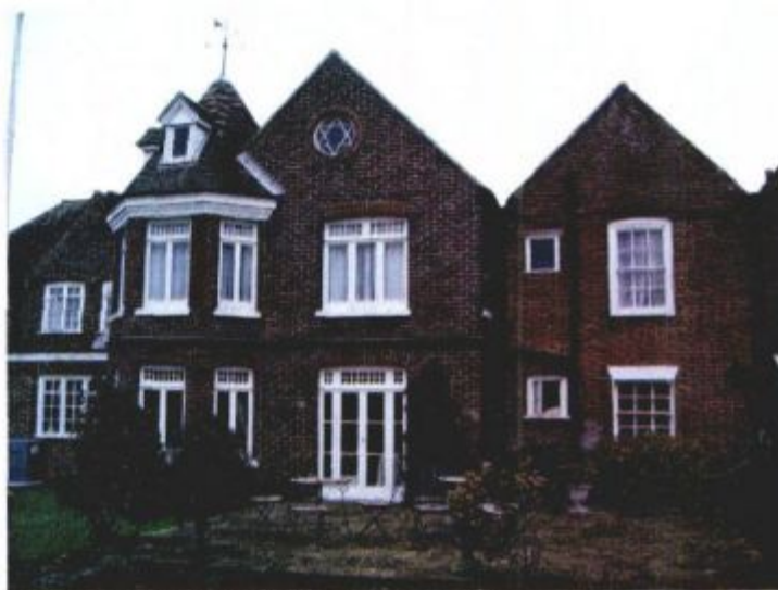
2.1 West elevation showing existing terrace
