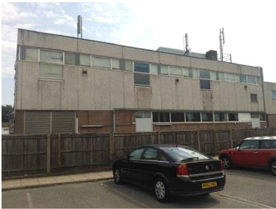
PHOTO OF NORTH WEST ELEVATION
