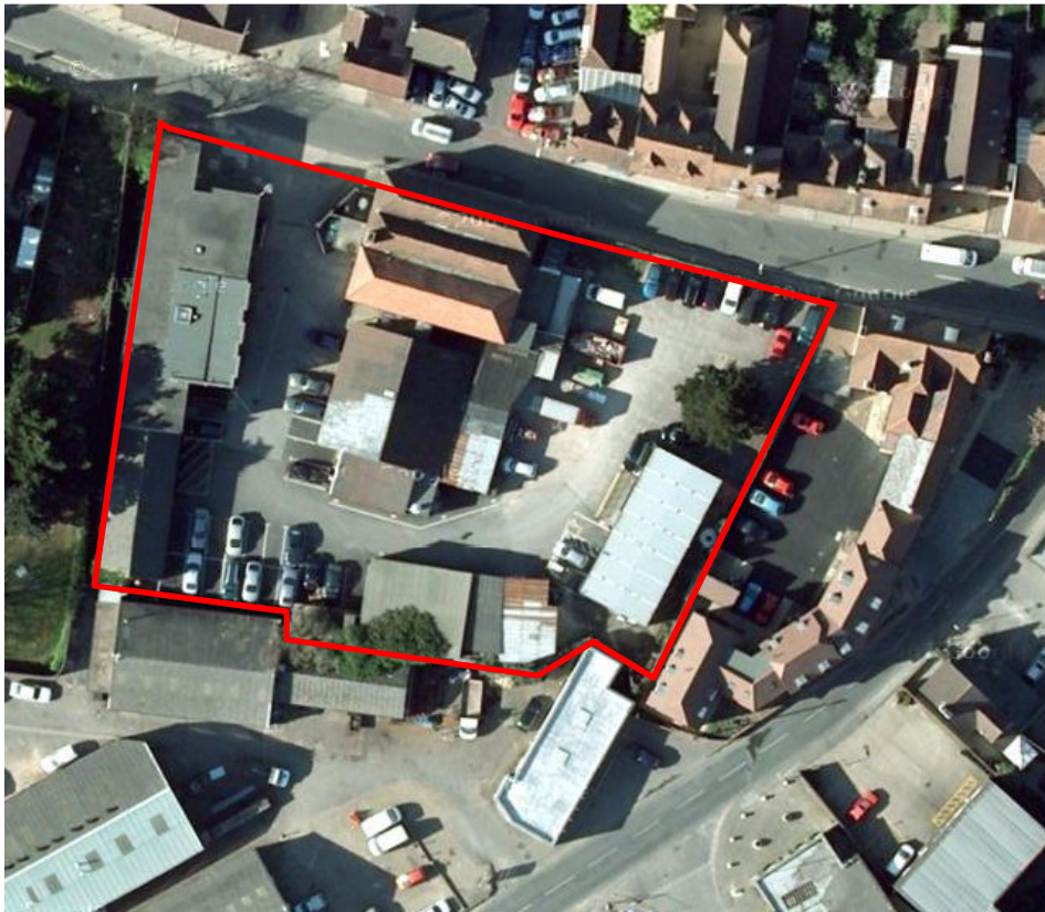
Aerial view on site
