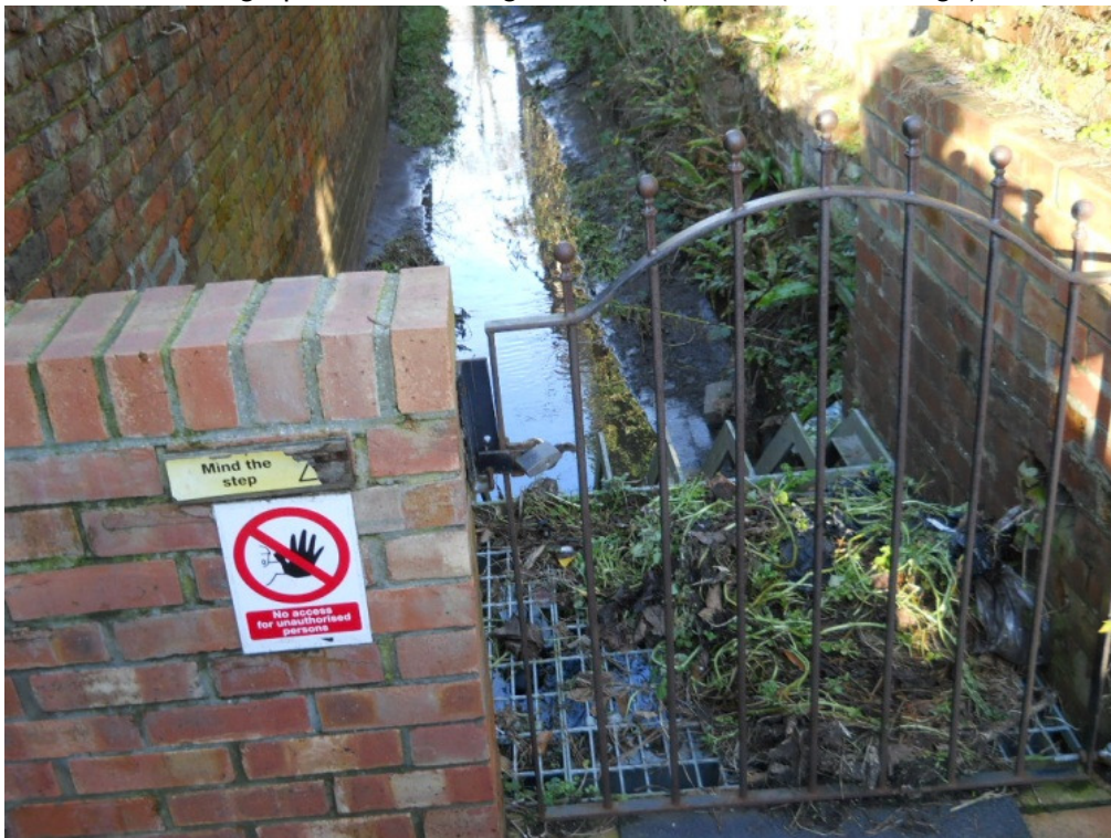
Trash screen adjacent SW corner of site
