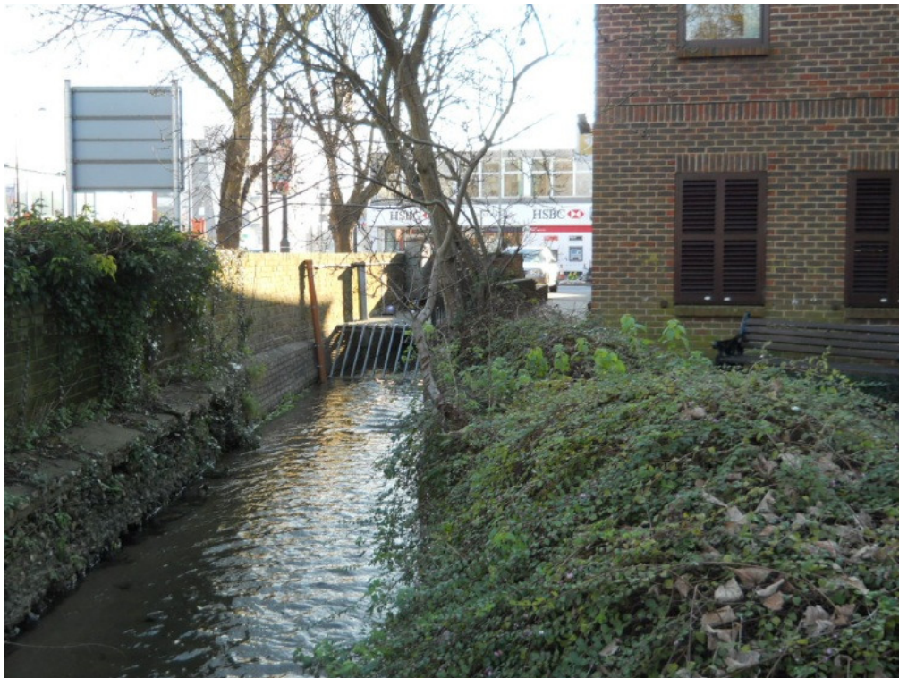
Main channel and trash screen below offtake and just upstream of West Street
