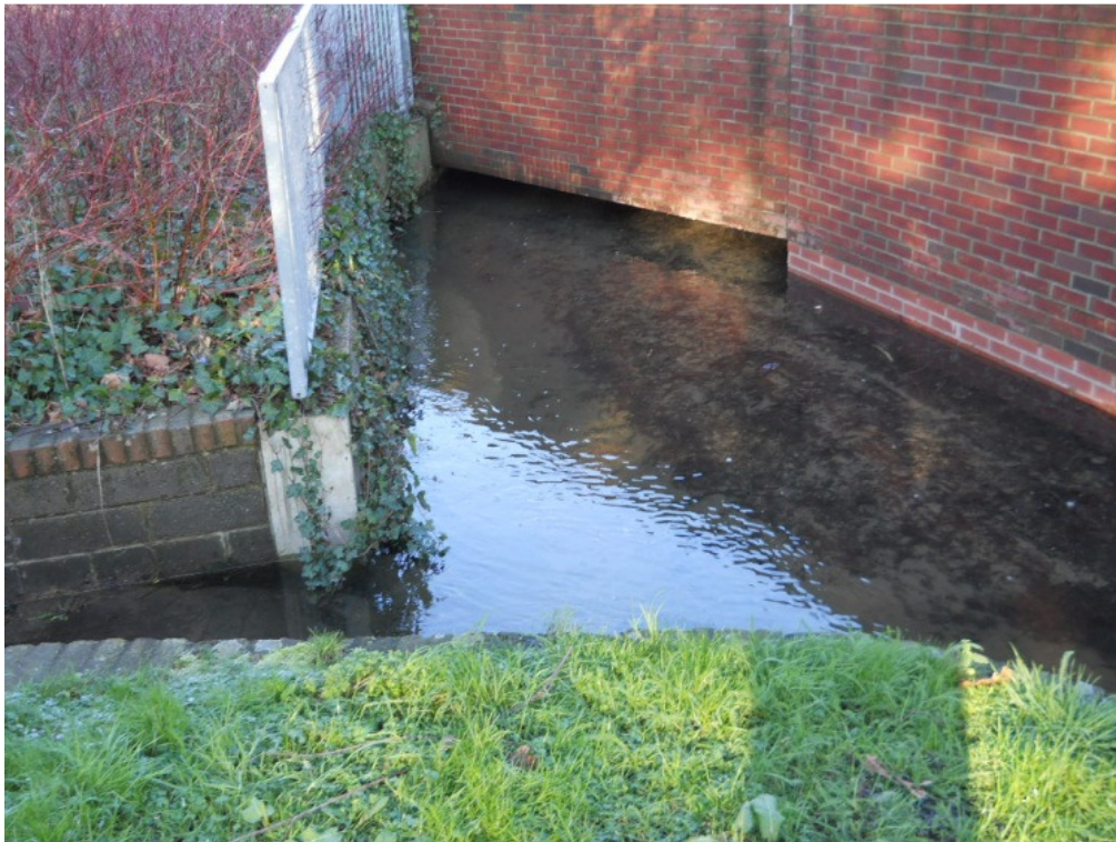
Mill race off take(LHS) from main channel
