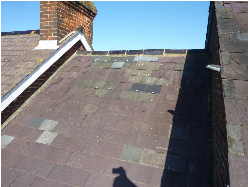
View of roof above first floor over garage.
