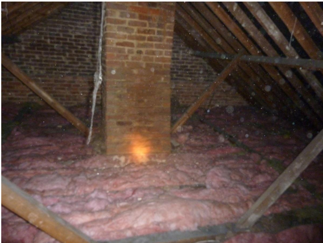
Roof void with hanging cobwebs .
