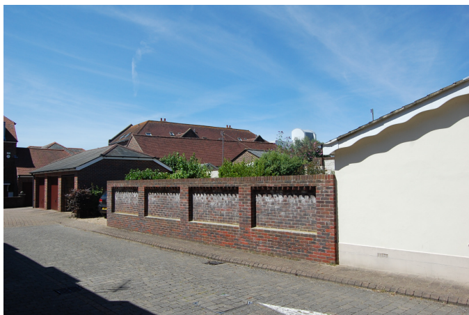
Site garden wall along Stanley Road
