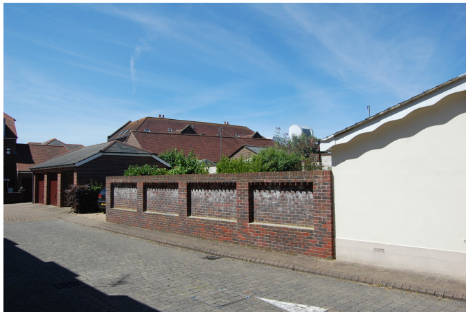
Site garden wall along Stanley Road to be replicated for rear garden boundary
