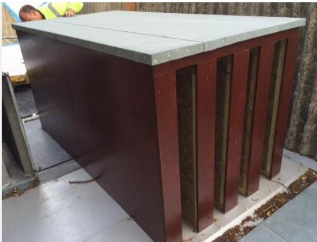
Enclosure with Splitter Outlet Attenuators
