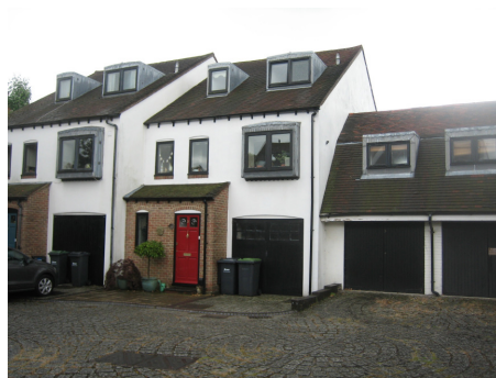
Fig 1 – Front view of the property within courtyard
