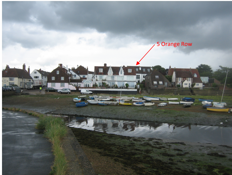
Fig 4 – View of property from millpond footpath
