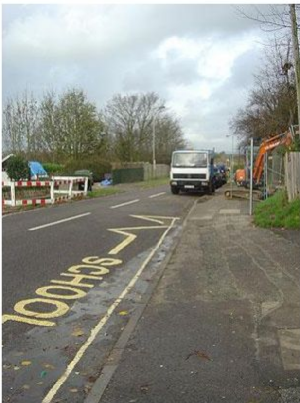
Front Entrance to School looking North
