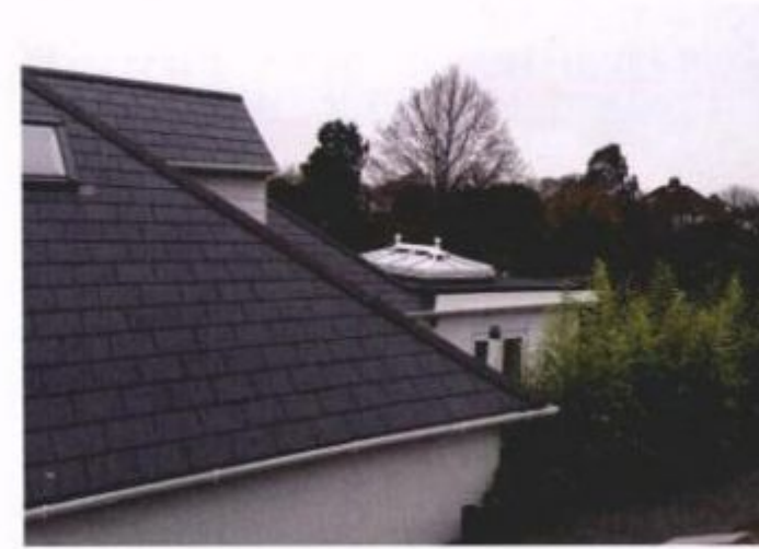
Existing photograph, north east overlooking neighbouring rear garden
