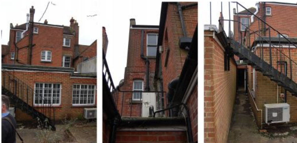
Images of the rear of the building
