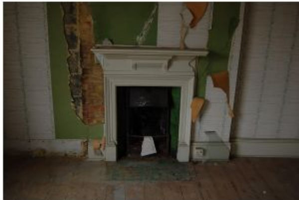
Strong feature fire place. Second Floor.
