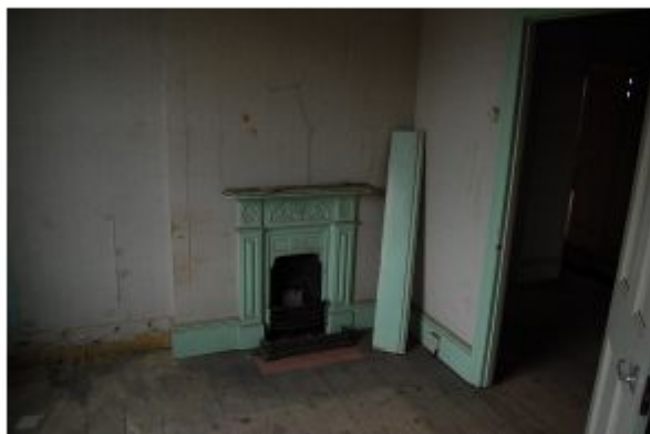
Fire place that will be located in Kitchen. Second Floor.
