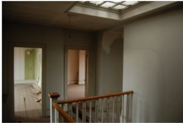
Balustrade to stair of good design. Second Floor.
