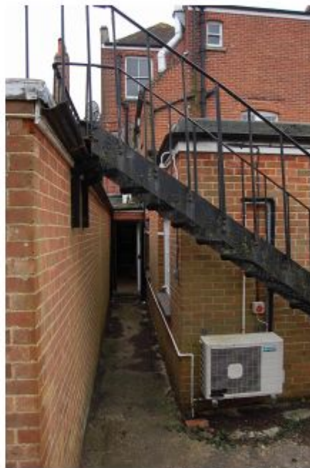
Fire escape removed. Not a part of historic character.
