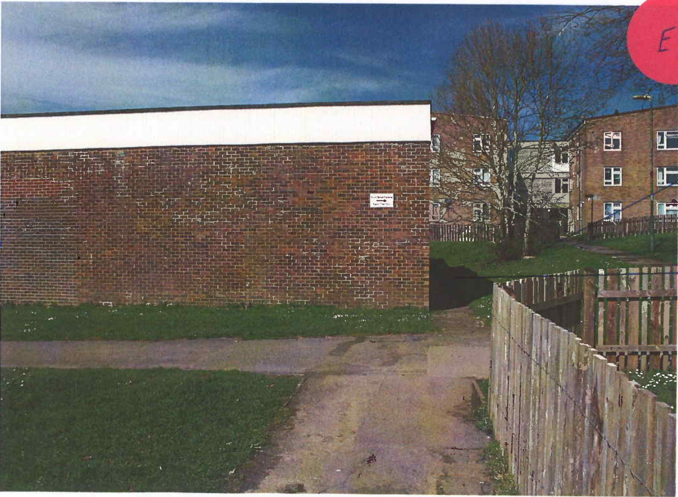
End view of Pre-school and adjacent land to be enclosed where new Gate will be
