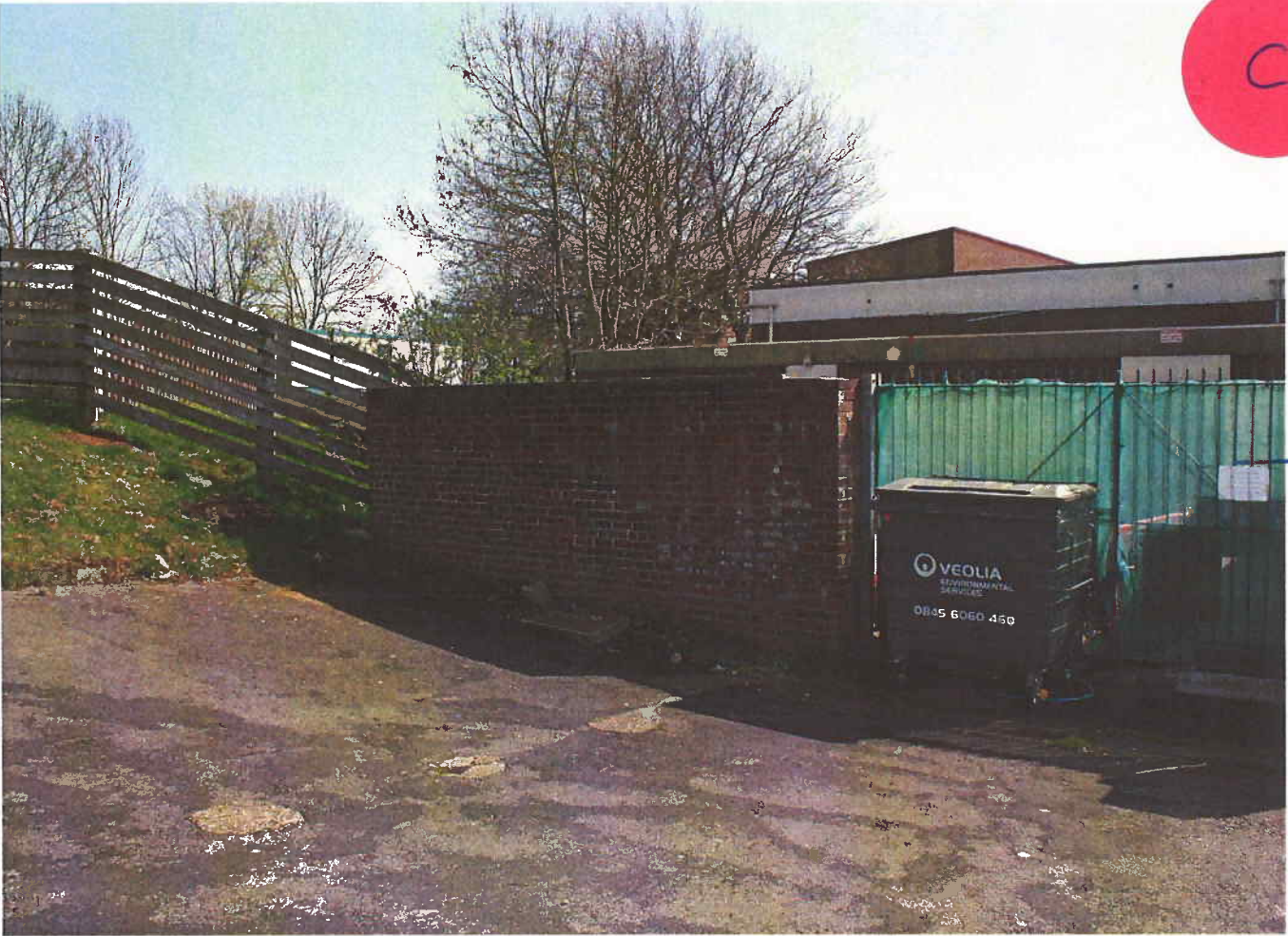
External View- REAR- of Wall to be removed and replaced by Fencing
