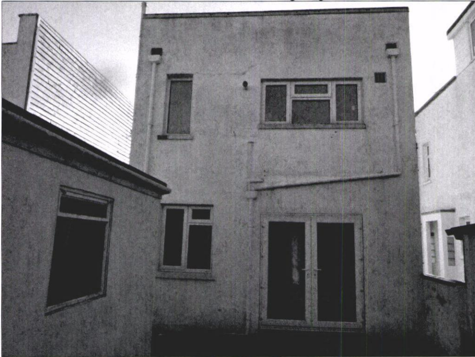
Rear of the house and garage.
