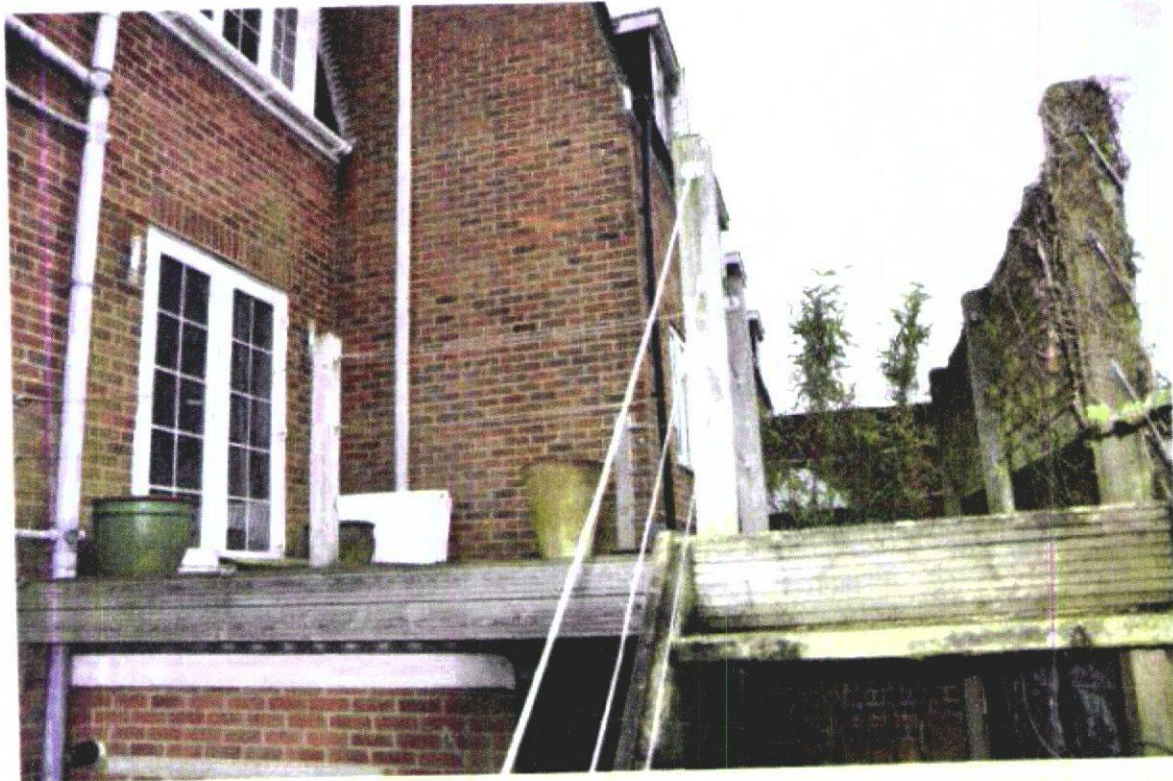
SNILE STREET - EXISTING BALCONY
