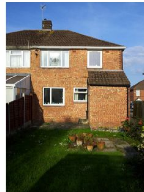
PHOTO REAR ELEVATION
