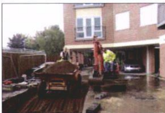
Photo 53: Structural tree soil retains sufficient structure for tree roots to grow, even when compacted.
