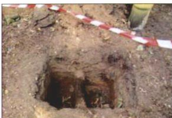
Photo 38: Where piles are proposed close to trunks, it is essential to excavate 50–75cm deep to see if there are any significant roots in the way, with provision to move the pile location if roots are found (note the pile was finally installed to avoid this root).
