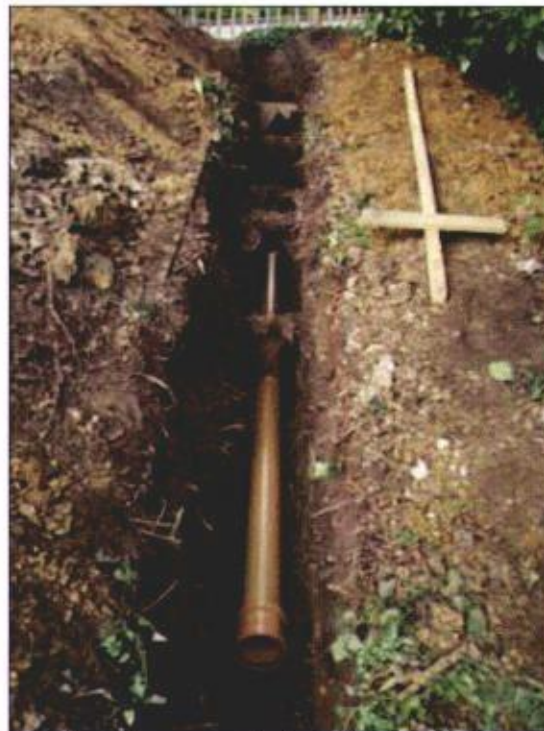
Photo 45: Continuous trenches dug by hand so that important roots can be retained (with the service ducting threaded beneath) is an effective means of minimising damage (note the ground protection boards with soil piled on top on the left).
