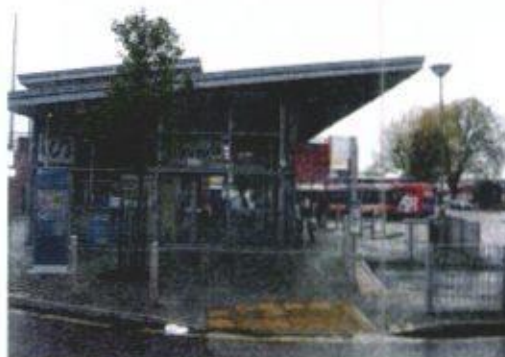
Figure 3.7: Havant Bus Station
