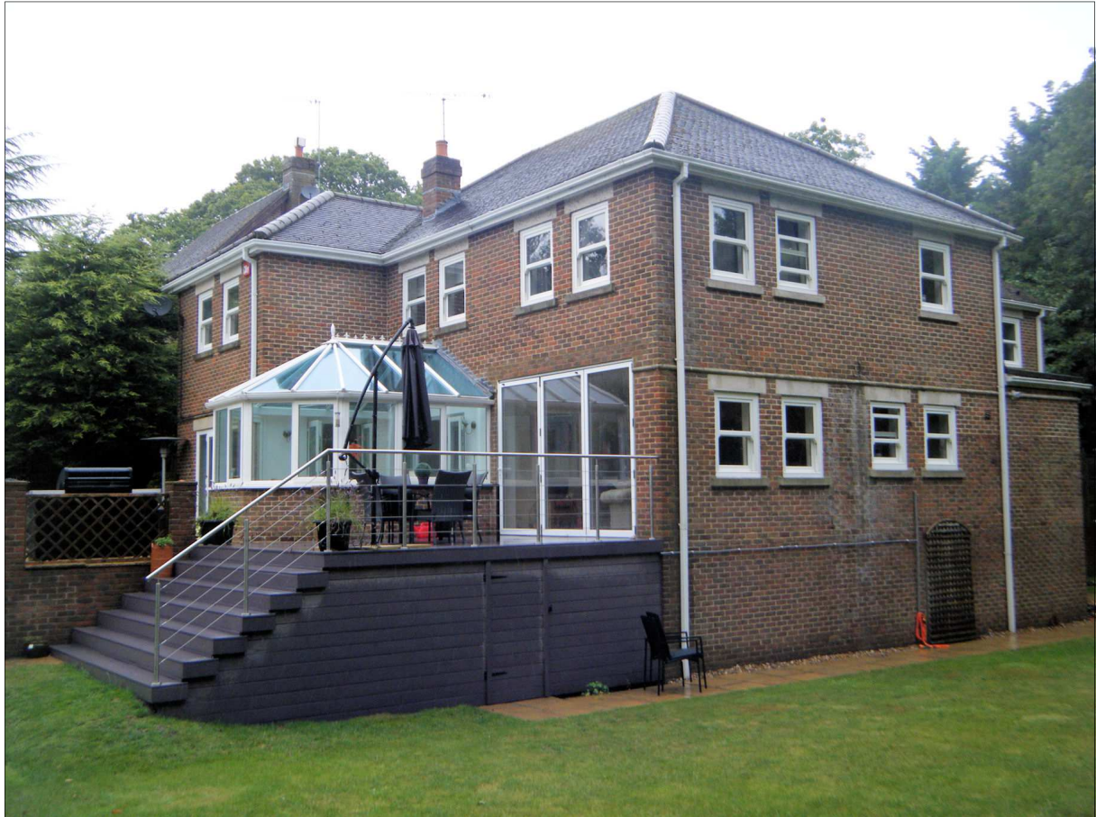
Rear and side view of No. 17 Billett Avenue
