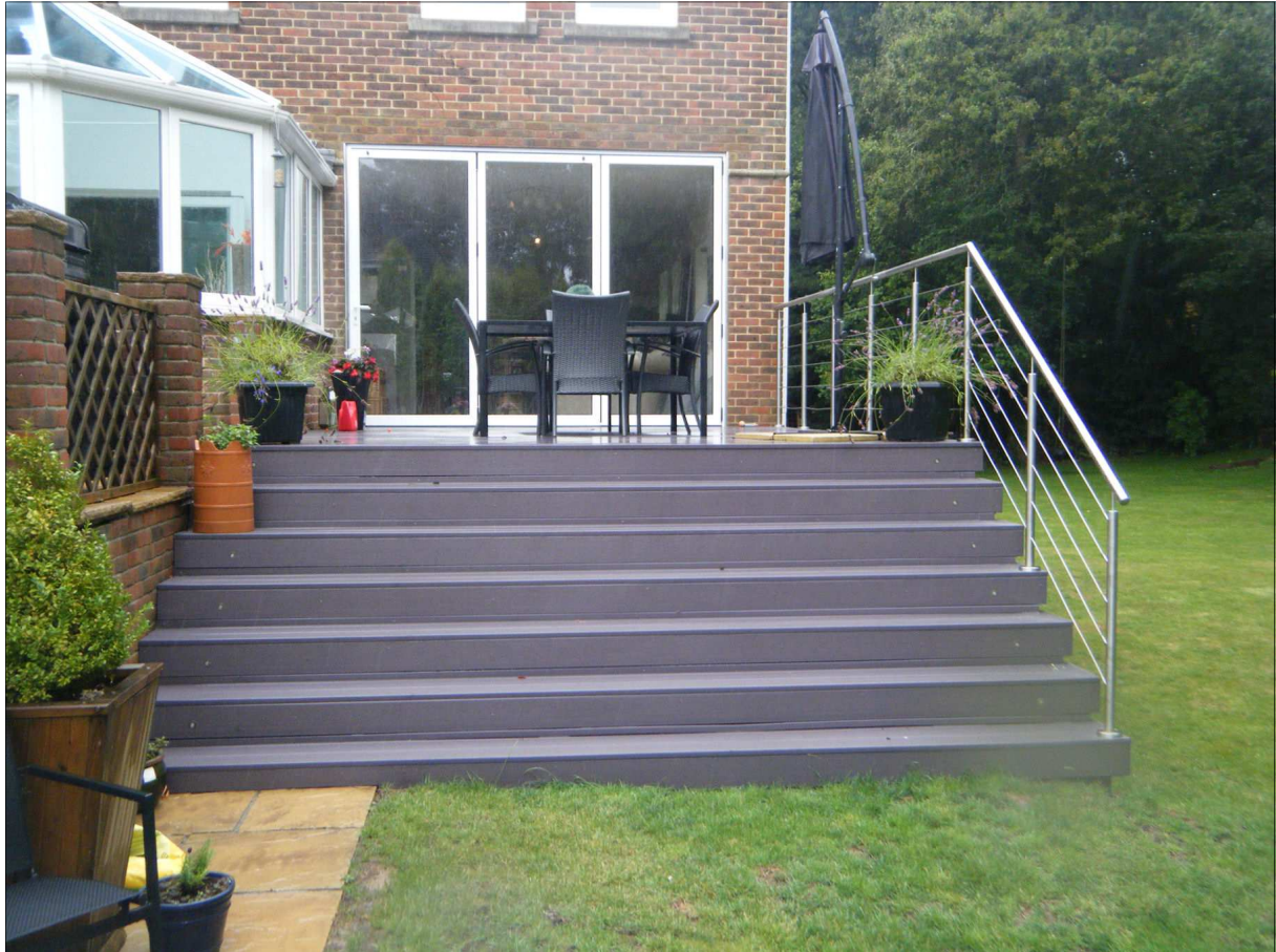
Side view of steps at No. 17 Billett Avenue
