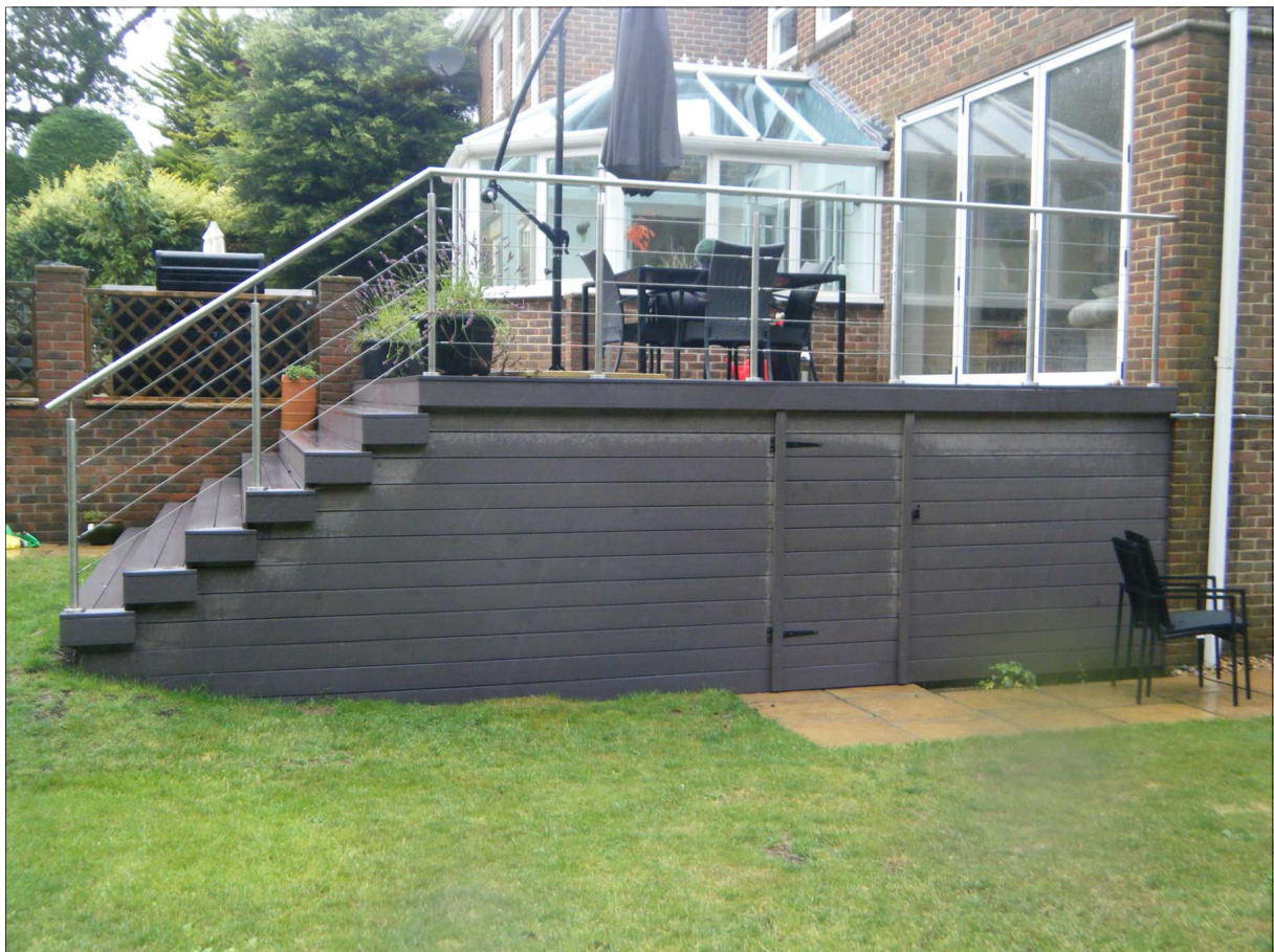
Rear view of steps at No. 17 Billett Avenue
