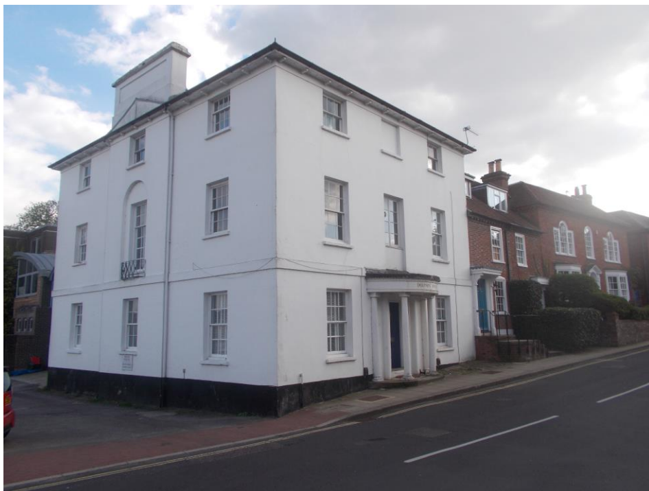
Figure vi. 29 Queen Street and adjacent listed buildings Nos. 25 and 27 to the west of the site.
