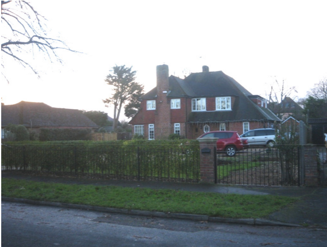
19, Castle Avenue looking towards no 15
