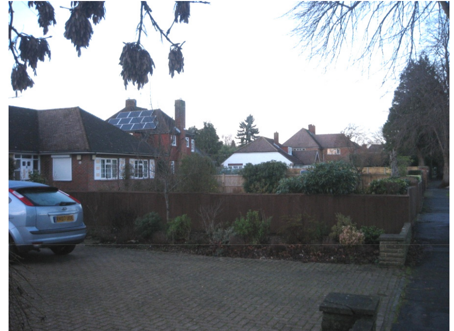
View of 19, Castle Avenue from the front of no 13 showing no 15 in the foreground and nos 21 and 23 beyond.
