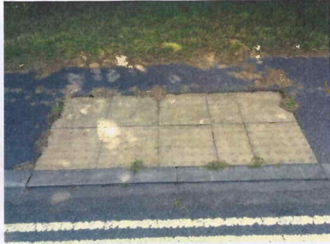
Photographs showing lack of maintenance observed at the crossing points.
