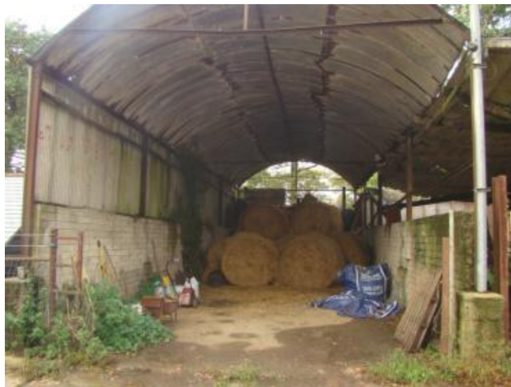
Figure 7: Barn where switch room is attached externally
