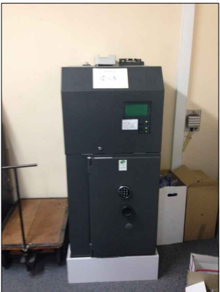
External ATM - Internal View
