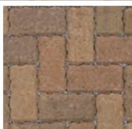
Driveline Piora, Bracken (BRA)
