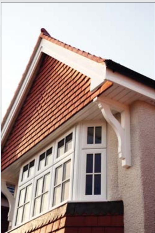
Photo 5 : Tile hung gable end
