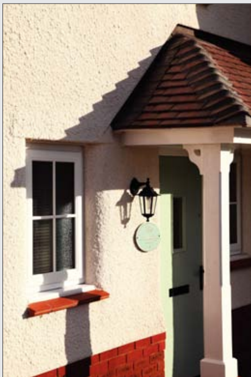
Photo 8 : Timber post porch
