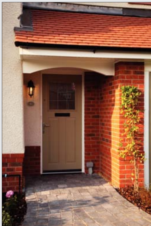
Photo 8 : Tile roof porch
