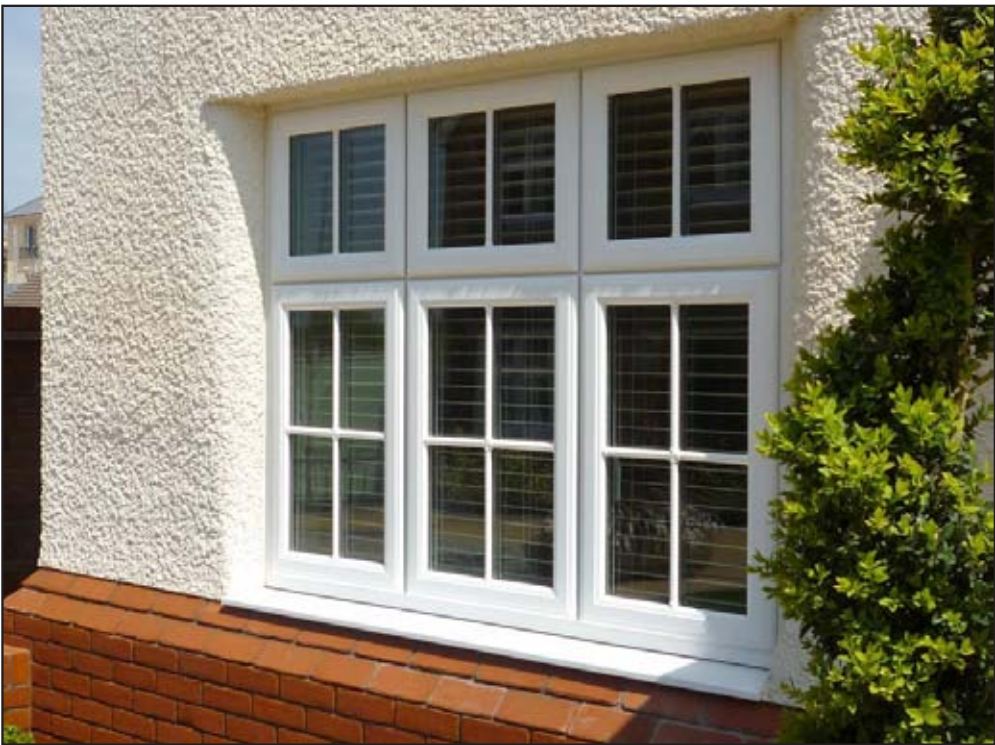
Photo 2 : Roughcast white render rounded into the window reveal
