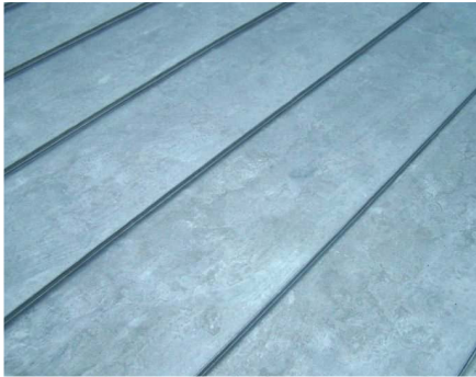
Standing seam zinc roof
