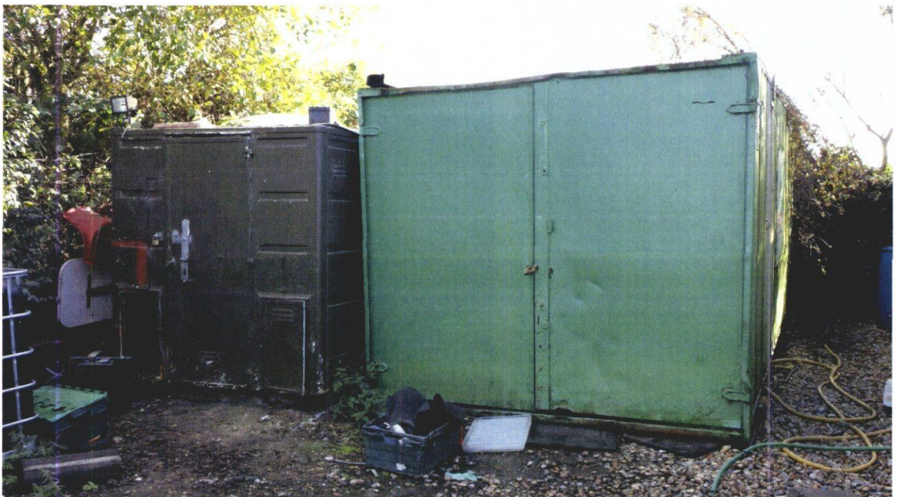
STORAGE CONTAINER (LEFT) AND GENERATOR CONTAINER (RIGHT):
