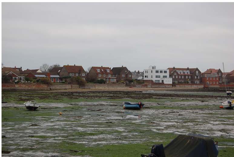
Line of rear elevations of neighbours
