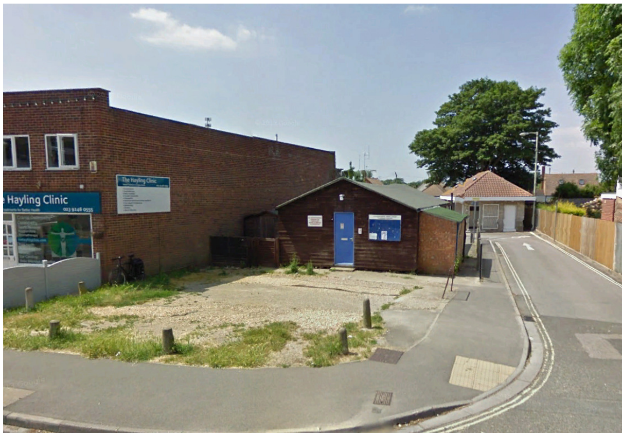
Front elevation of site
