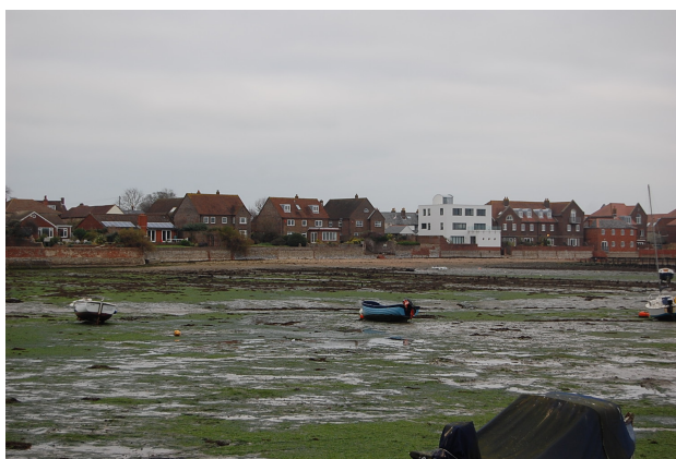
Line of rear elevations of our site and neighbours
