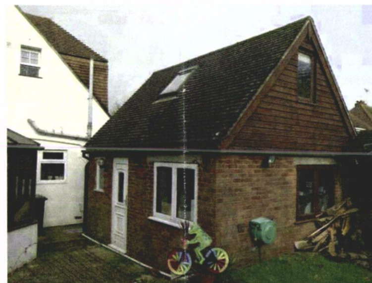
REAR VIEW (SOUTH / E)
