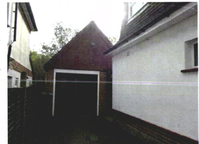
SIDE VIEW (EAST)
