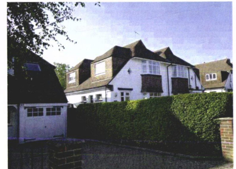
FRONT VIEW (NORTH / E)
