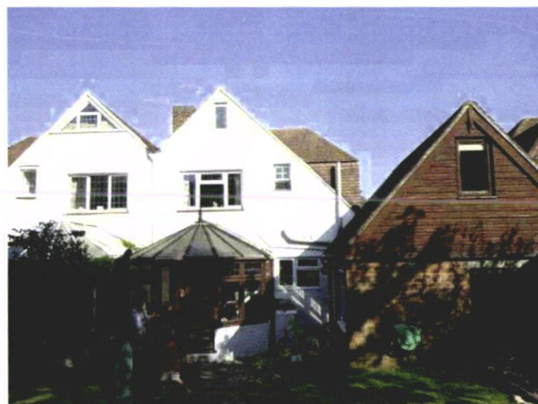
REAR VIEW (SOUTH)
