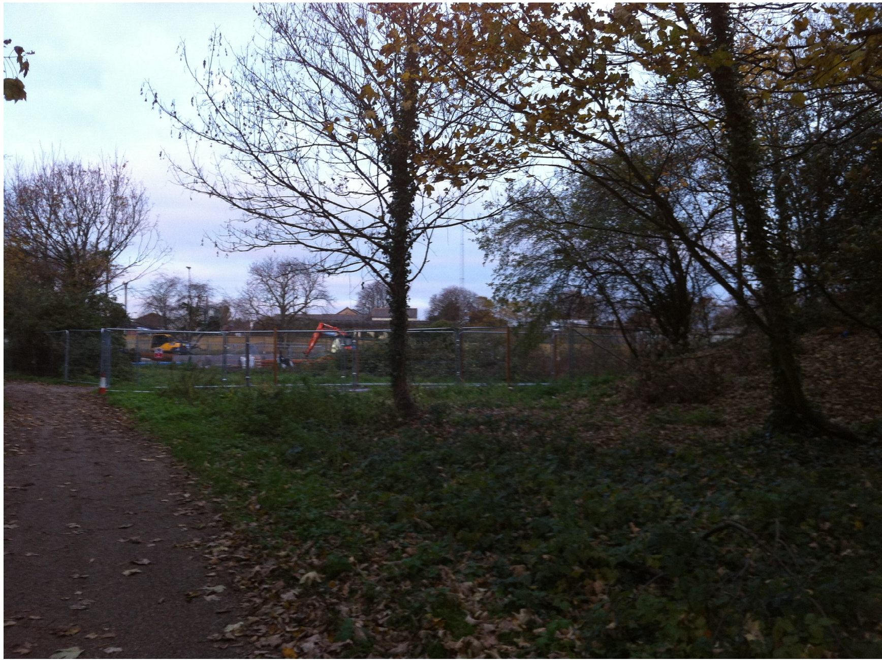
Current view to the north viewed from the centre of the Hayling Billy path perpendicular to the application site. Current under construction where Bloor Homes are about to construct 3 stoery properties facing towards the path
