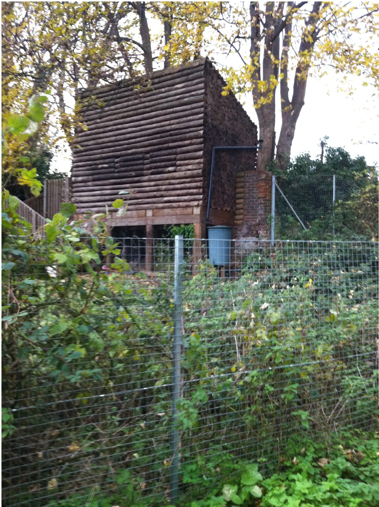
Photograph of the Hide which is believed to be to the rear of Fairfield School. Although wildlife may accept it's precence as undisturbing, is of camparative size, height and materials to the proposed extension of the garage and indeed offers a much greater visual addition than the proposal when viewed from the Hayling Billy path
