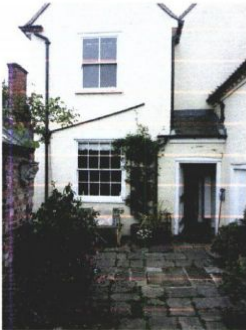
Rear section where extension will sit.
