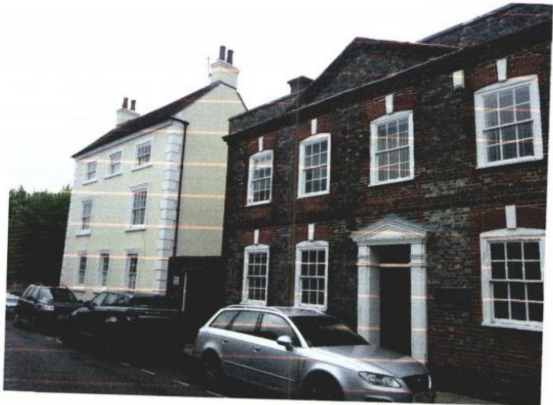
View of Front Elevation [Stucco Building to the left hand side of Picture]
