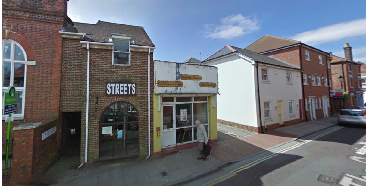
View of site from The Pallant
