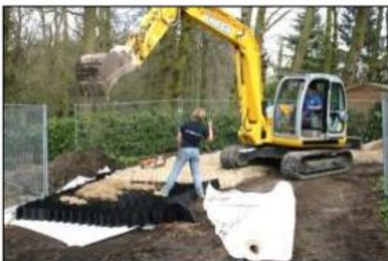
Photo 11: Cellular products are a very effective means of providing ground protection where heavy vehicle use is expected.
