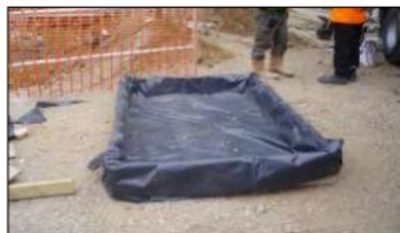
Photo 47: Soil bunding or a supporting framework covered in heavy-duty plastic sheeting is essential where there is a risk of spillages contaminating RPAs.
