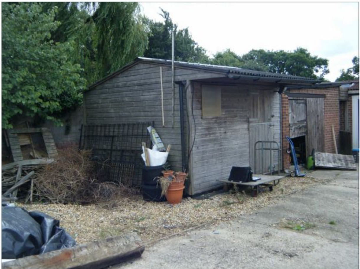
One of the outbuildings to be demolished
