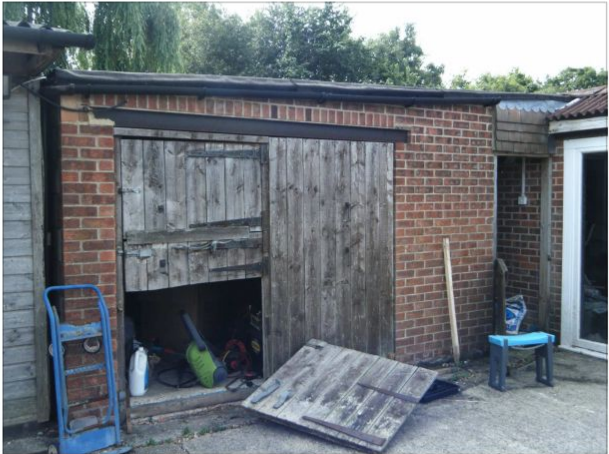
One of the outbuildings to be demolished
