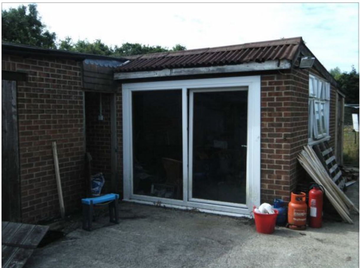
One of the outbuildings to be demolished
