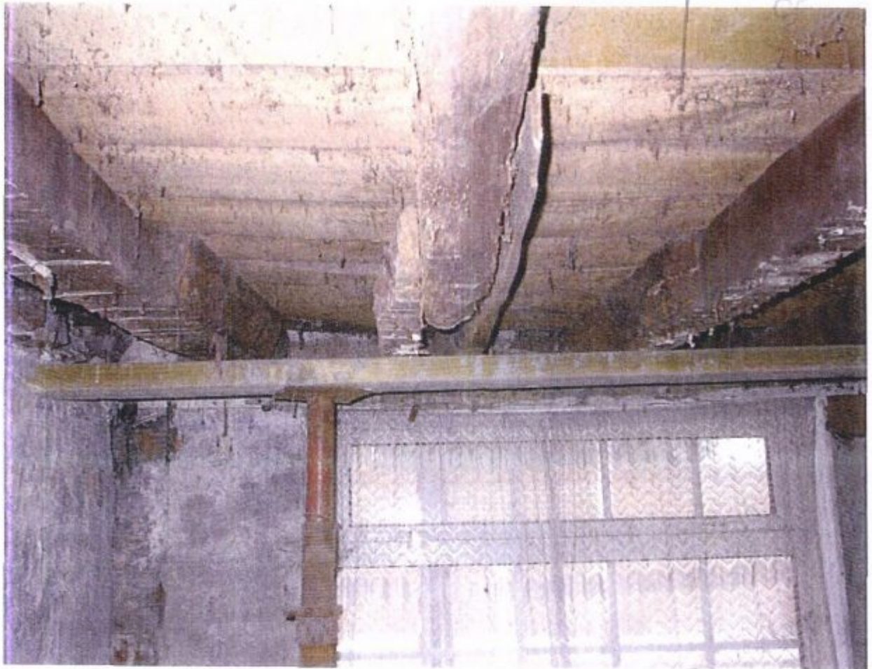
Photo No. 51 – Study:- 1 st Floor Joists.
