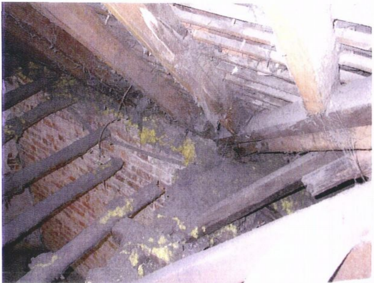
Photo No. 11 – Bedroom 3. East Ceiling Joists at Junction with Rafters.
