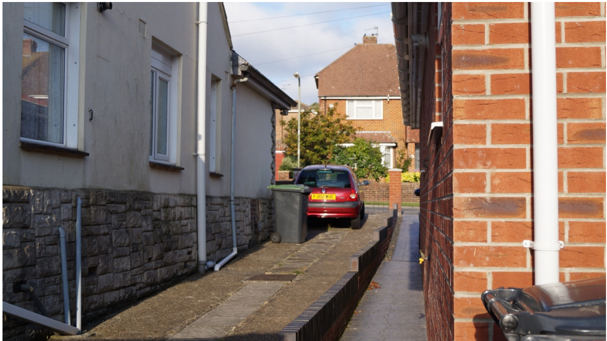
FIG 3. Rear Elevation of No. 200 (on the right) - Image taken 21st September 2014 at 08:37am. No Overshadowing from No. 200 affecting No. 198.
