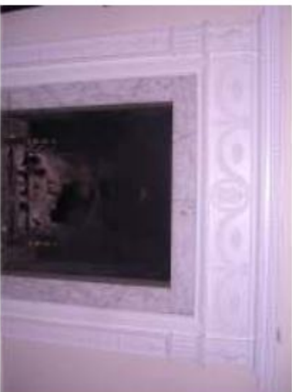
f - existing fireplace detail. (to be retained).
