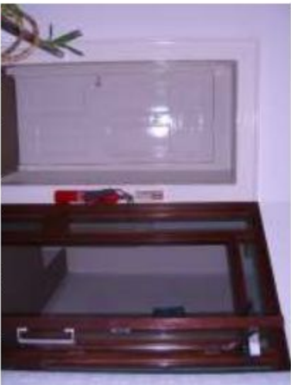
e - looking towards the partitioned wall for fire compartmentation which will be removed
