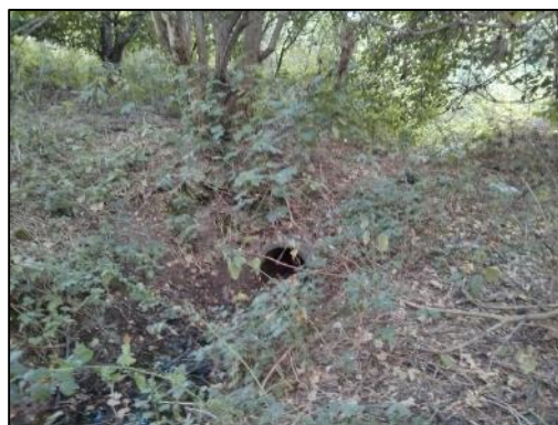
Figure 4: Culvert near the centre of the northern boundary of the site
