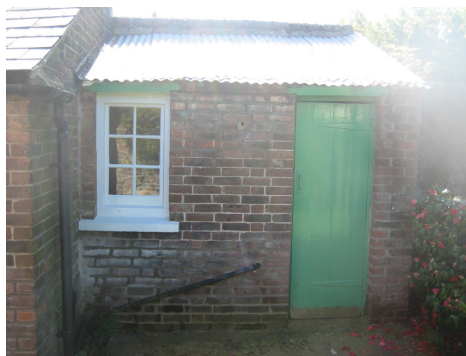
Fig 3 – View of existing outbuilding from rear garden
