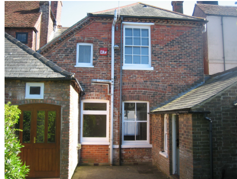
Fig 2 – Rear view of property.
