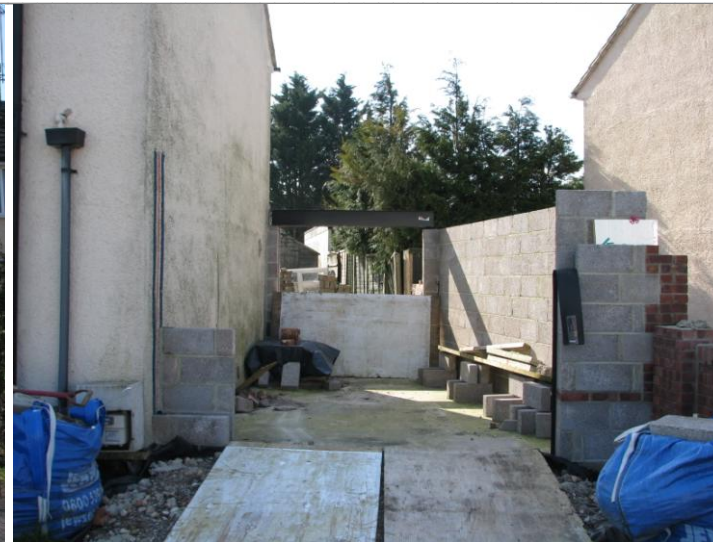
Above: Front Elevation of Partially Complete Garage
