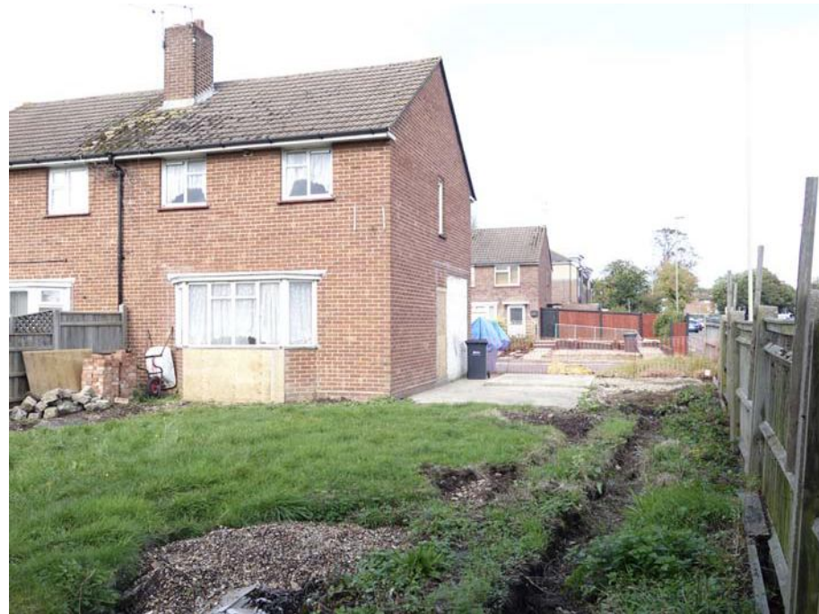
REAR VIEW (SOUTH EAST)
