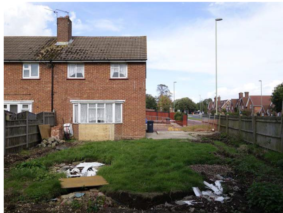
REAR VIEW (SOUTH)
