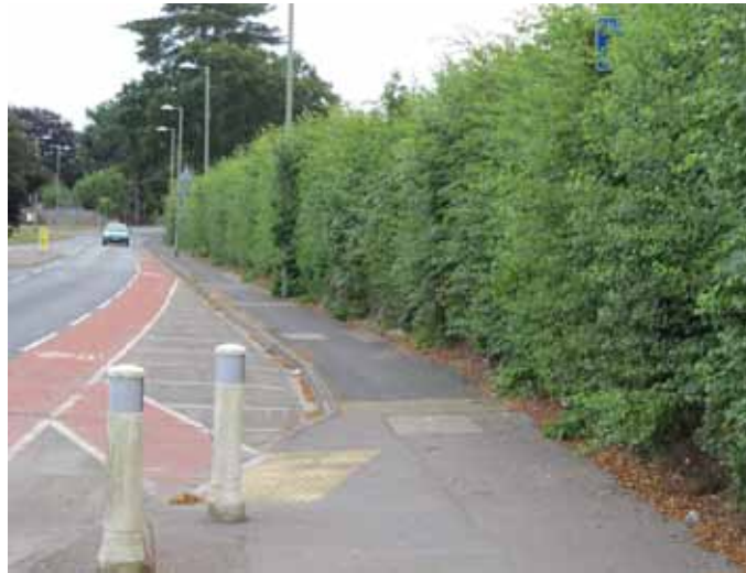
SOUTH ALONG HORNDEAN ROAD
