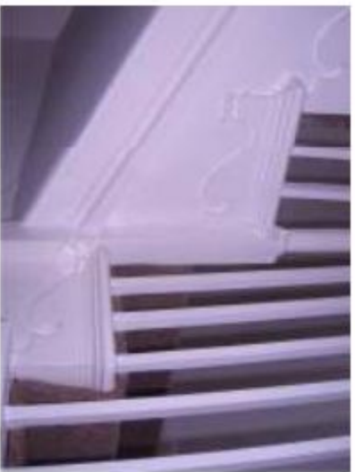
staircase detail (from photo-g)
