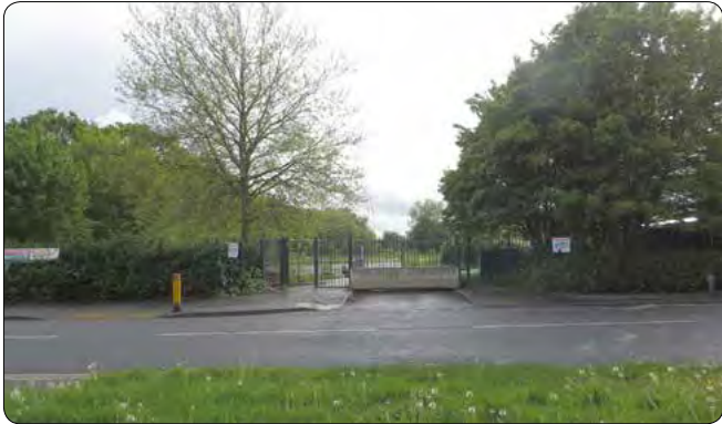
B. View into site entrance
