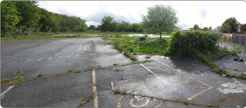
C. View into site
