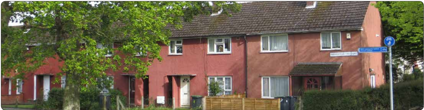
Priorsdean Crescent terrace housing
