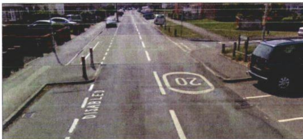
Figure 5.4 – Informal crossing facilities on Bramdean Drive.
